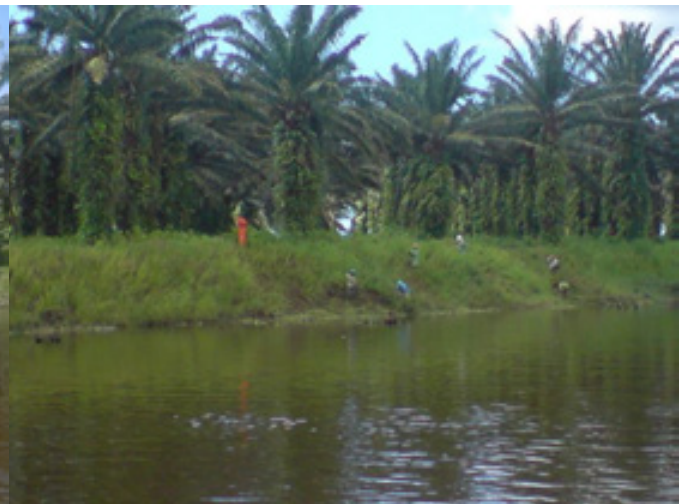
2 200 m Ivondro River bank Stabilized in 2009
