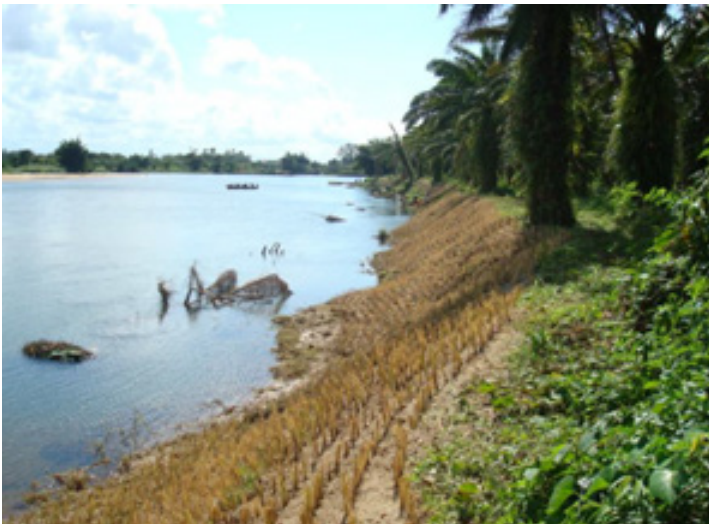
Trying to protect river bank by Vetiver
